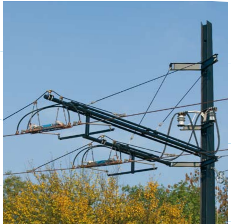
Sectioning with four feeders
