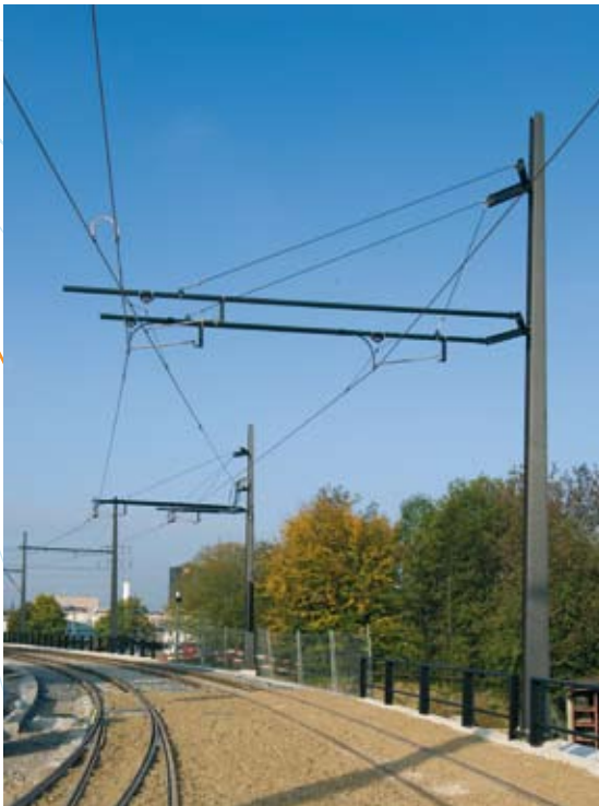
Twin cantilever over turnout
