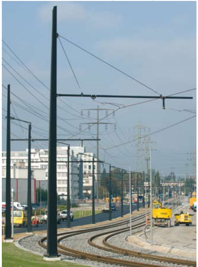
Combined registration and support on curved track
