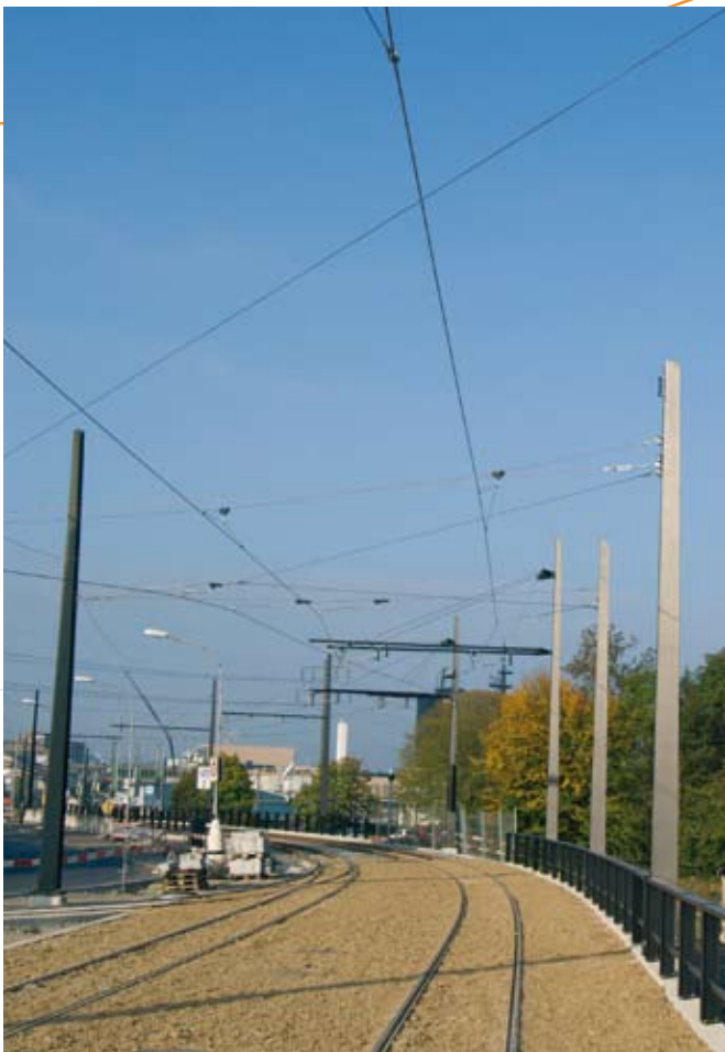
Cross span with delta cable suspension
