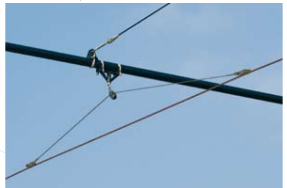
Delta suspension with pulley
