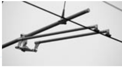
Single or double steady arm with contact wire
