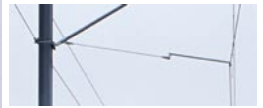
Flying steady arm pull-off
