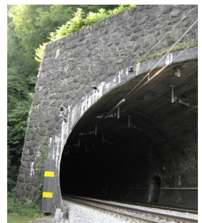
Tunnel with conductor bar. Location: Kerenzerberg CH
